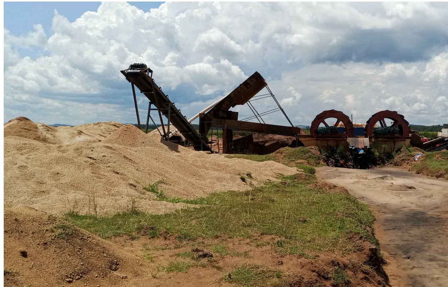
A sand mining site within Nakiyaga wetland system in Masaka District owned by Chinese investors .Nema ordered that the activities stop but the investors have continued to operate normally
